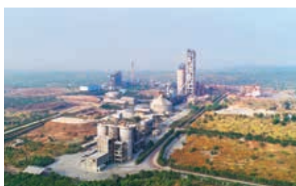
Sagar Cements (R) Limited Gudipadu, Andhra Pradesh
